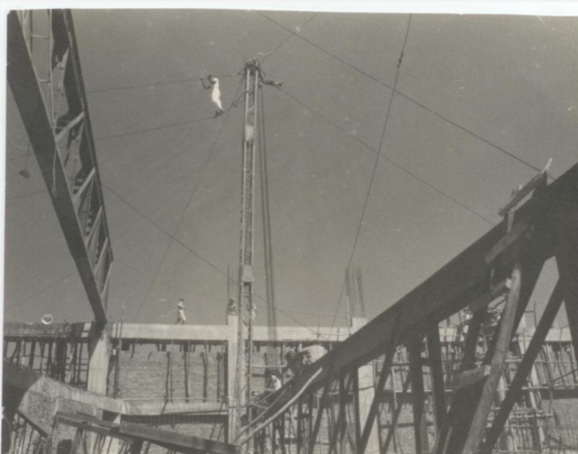
Construction of Homi Bhabha Auditorium
